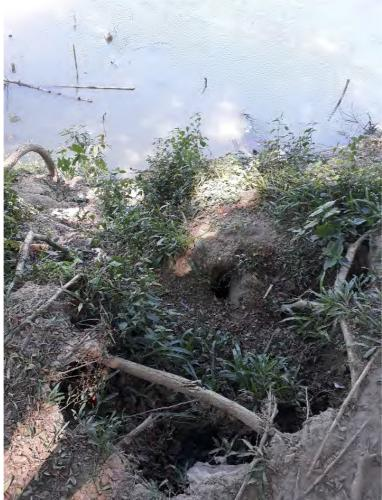
Photo 3 Scouring from surface water runoff on top of the riverbank
