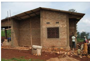
Administration building under construction
